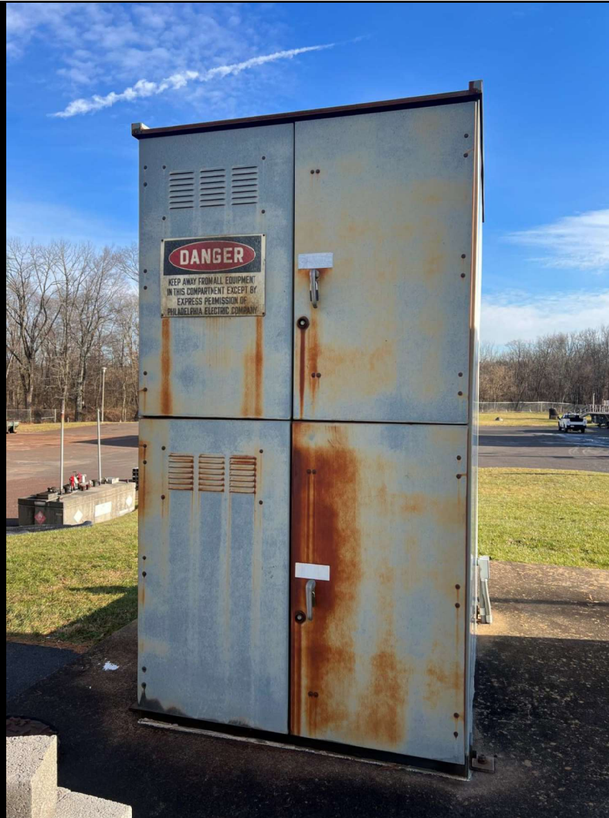
2 of 2 – 33,000 KVA Fuse Box
